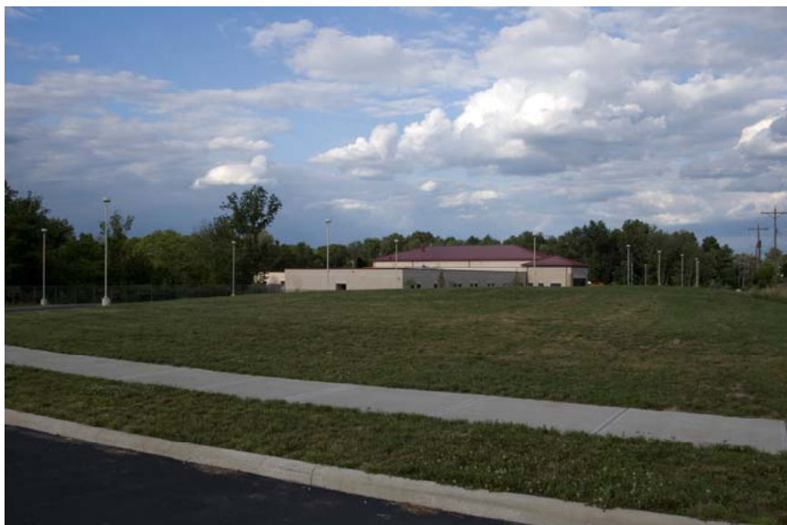
The new elementary school, East Linden, in the Arlington Park neighborhood.
